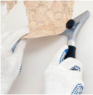
Remove previous wallpaper remnants or residues of old wallpaper paste.
